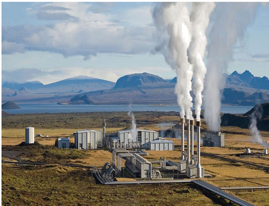
Iceland's Nesjavellir geothermal power station. Geothermal plants account for more than
